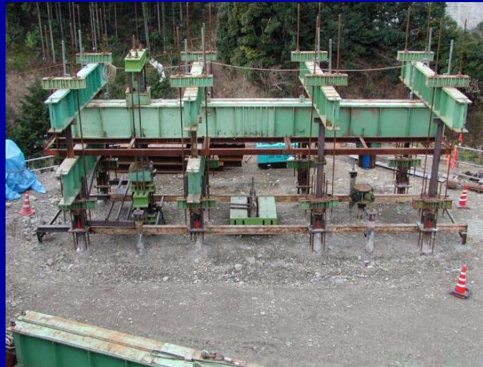
Full-scale field testing (Fujita Corp.)
